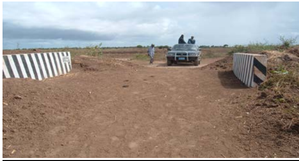
Culvert Box constructed
