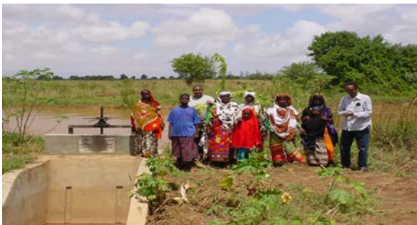
Sluice gate constructed
