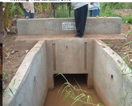
Culvert box constructed 2005
