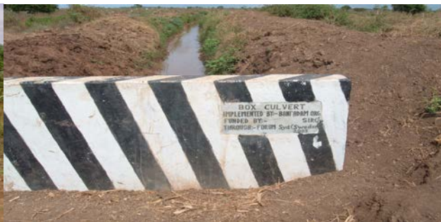
Number of culvert boxes constructed in 2003-2005 by SIRC-Baniadam
