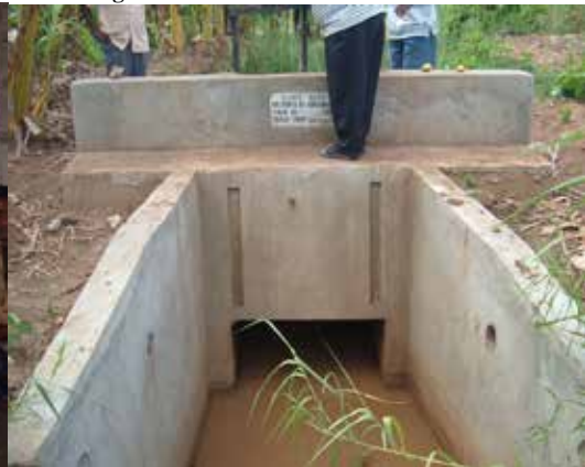
Culvert box constructed 2005
